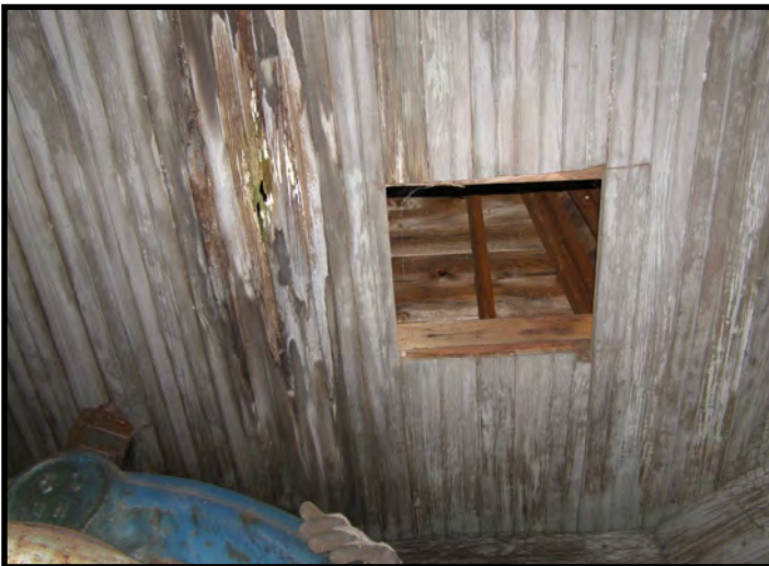
Steeple - Opening Between Bell Tower & Spire
