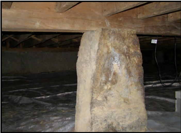
Granite Main Supports Beneath Original Building
