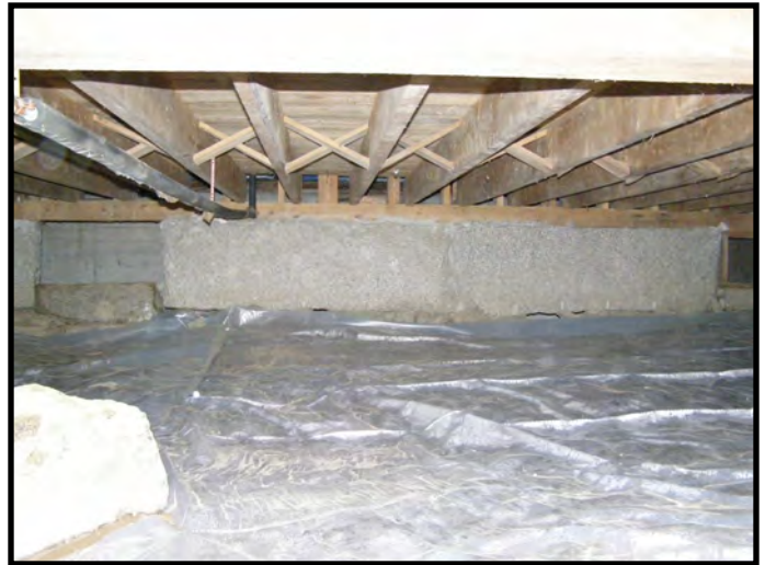
Beneath Original Building Looking Towards Salyards
