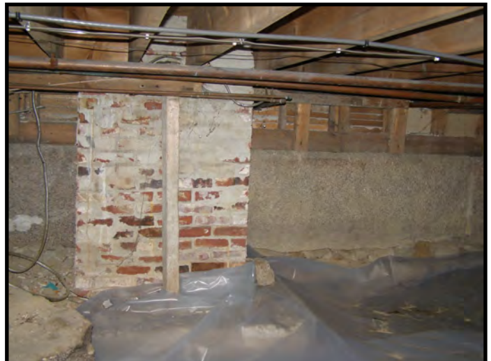
Base of Chimney - 1955 Crawl Area - Looking South
