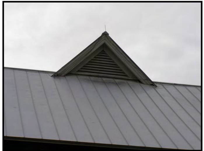
Exterior View - Operable Gable End Louver
