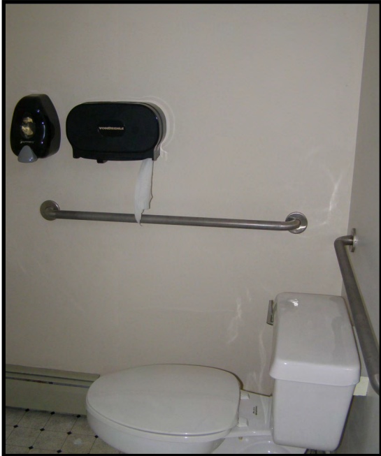
Fellowship Hall Restroom - Completely Salvageable
