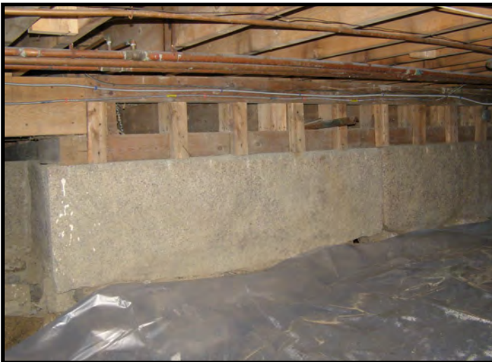
Foundation Beneath Original Building Area—North Side
