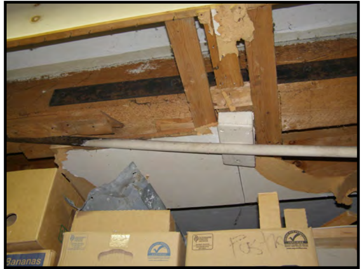
Tension Rod & Compression Block Beneath Sanctuary
