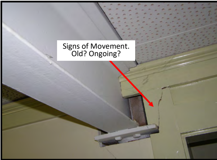
Wide Flange Floor Support Beam - Lower Hallway
