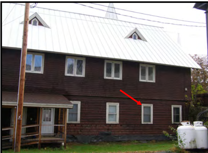
Partial View from West
