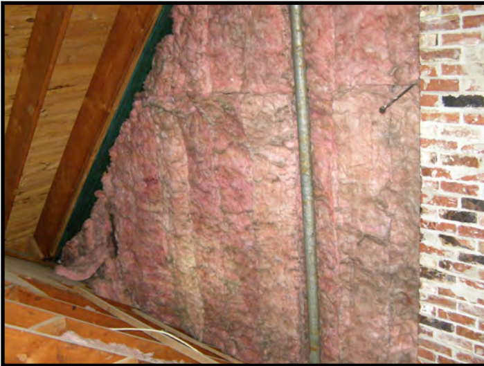
1955 Attic - Insulation of Original Building Gable End
