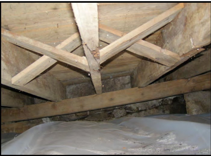
Floor Framing Beneath Main Entry - Looking East
