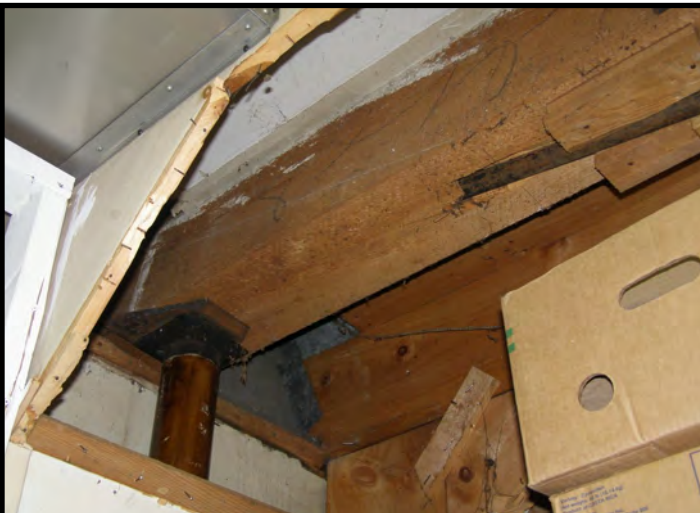
Column, Tension Rod & Main Floor Beam Beneath Sanctuary
