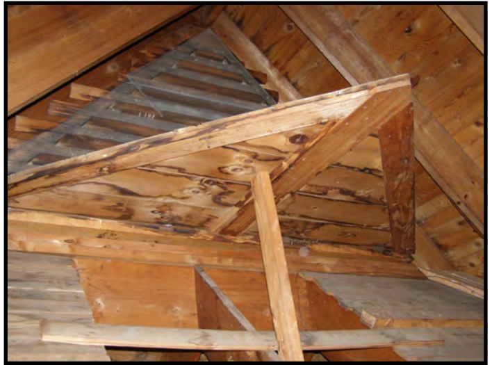
1955 Attic - Operable Gable End Louver at North End
