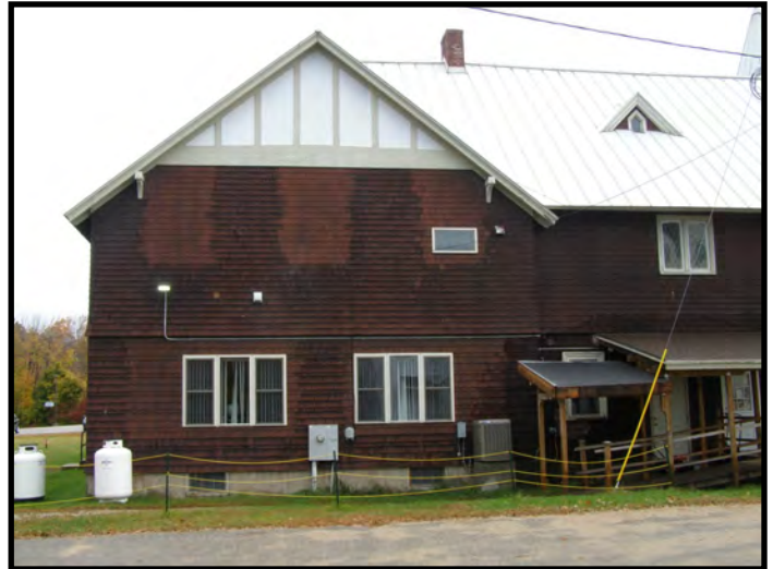
Partial View from West
