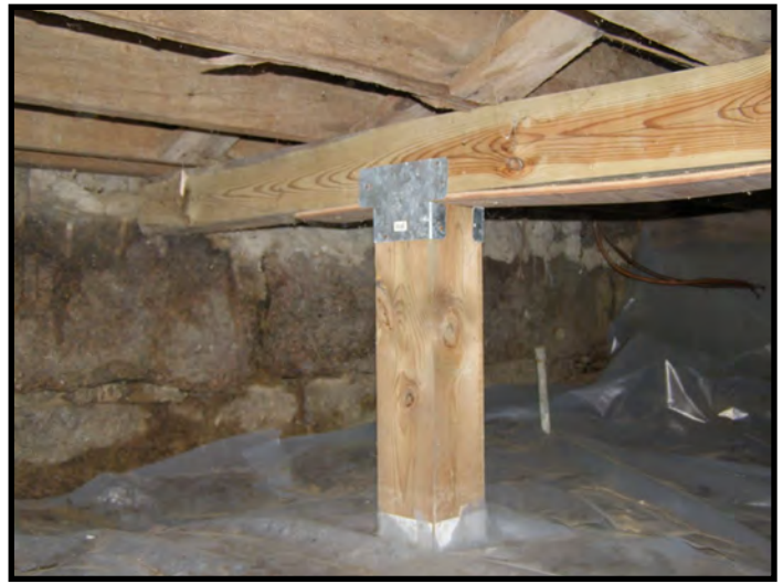
Improved Supports Beneath Original Building.
