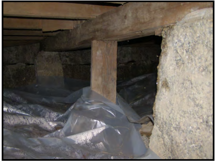
Additional Support Beneath Original Main Floor Carrying Beam
