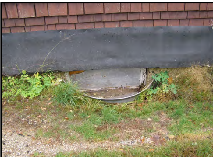
Abandoned Basement Window Well - Infill? Improve Drainage?
