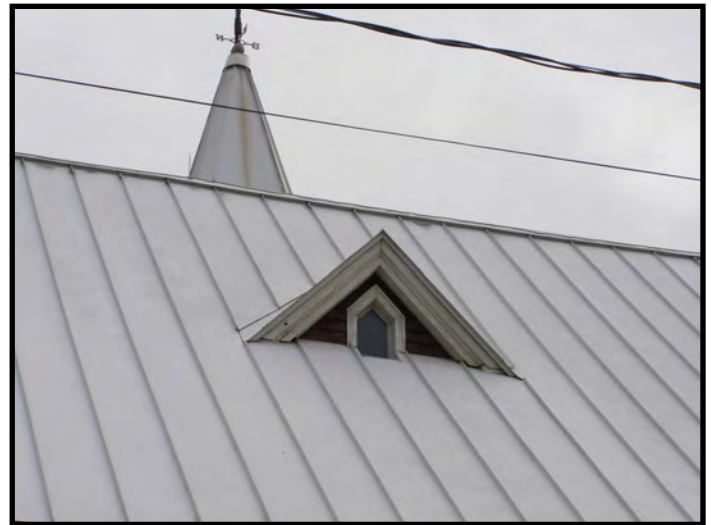
Small Dormer at Sanctuary - Completely Salvageable
