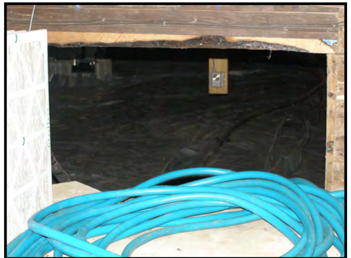
Opening, Mechanical Into Original Crawl Space
