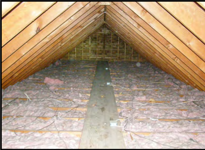
1955 Attic - Looking Towards Salyards
