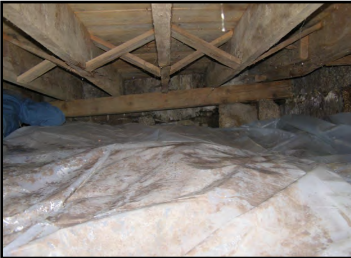
Beneath Main Entry Looking Towards Salyards
