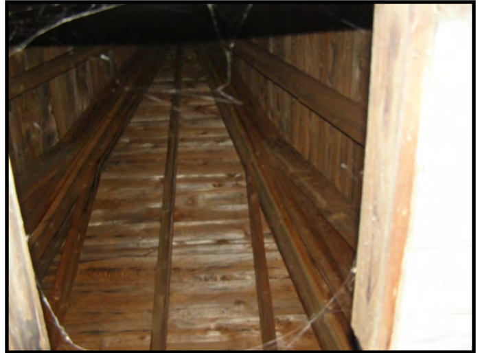
Steeple - Looking Upward Towards Spire
