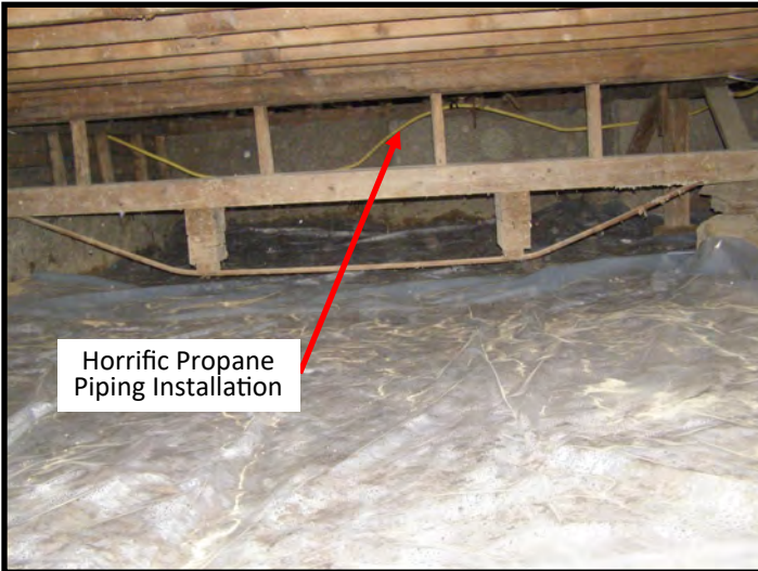
Beneath Food Pantry, Looking North Beneath Restrooms
